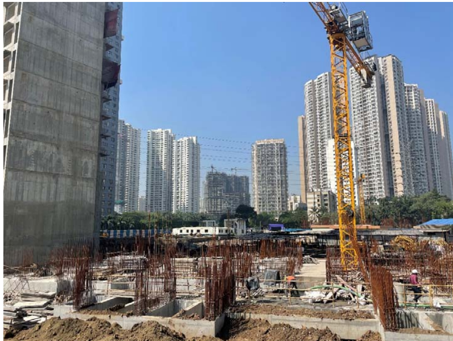
Tower – E Construction Status
