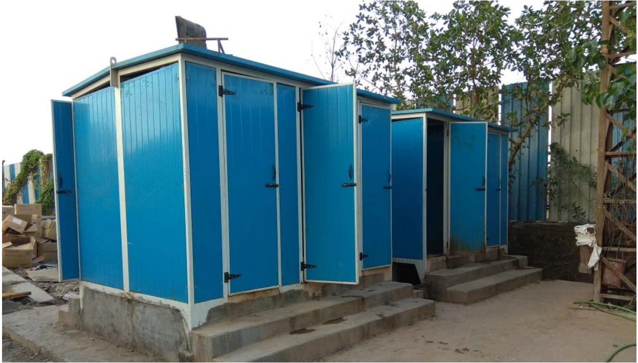
Toilet For Workers
